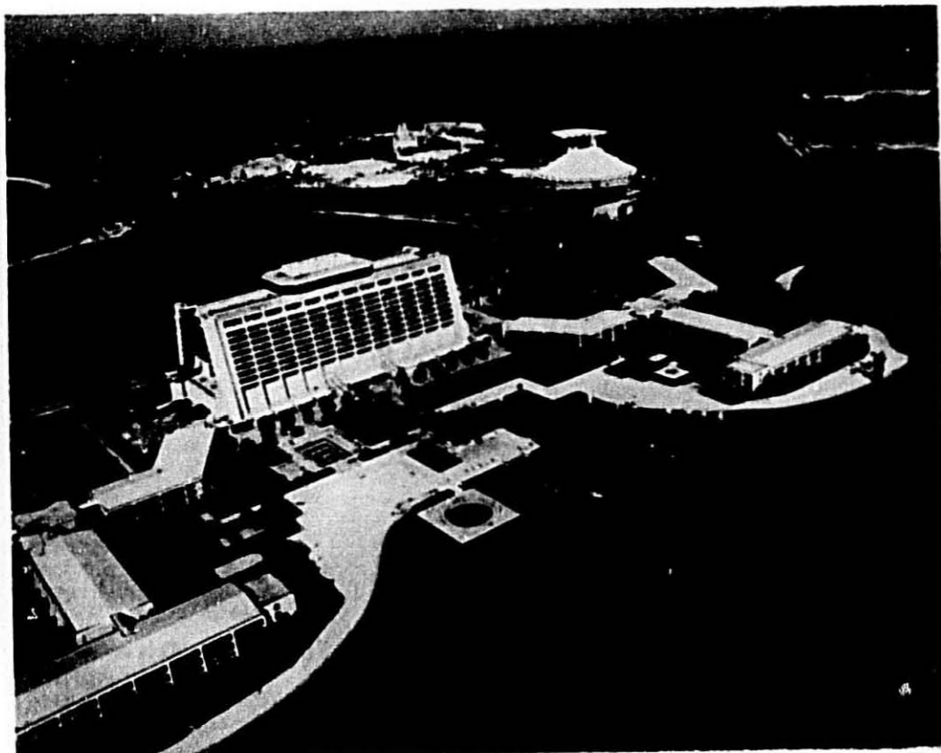
The Contemporary Resort Hotel rises majestically from the shores of Bay Lake. With sleek monorails running silently through the center of the A-framed tower building, the Contemporary Resort is a unique headquarters for visitors who dream of what a trip to the future might encompass.
